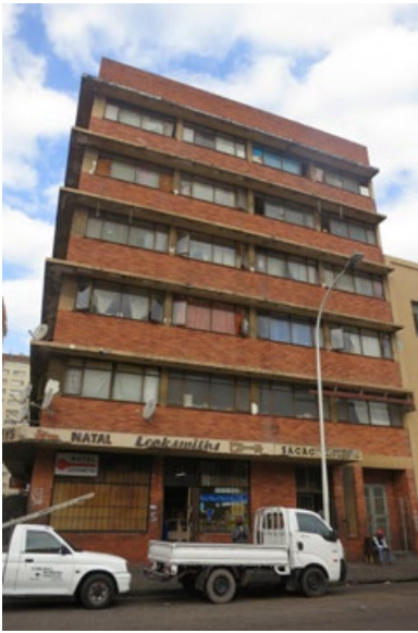
Fig. 10. A 2015 view of the former Security Branch police offices in Masobiya Mdluli Street, Durban. © Durban Local History Museums Collection, eThekweni Municipality
